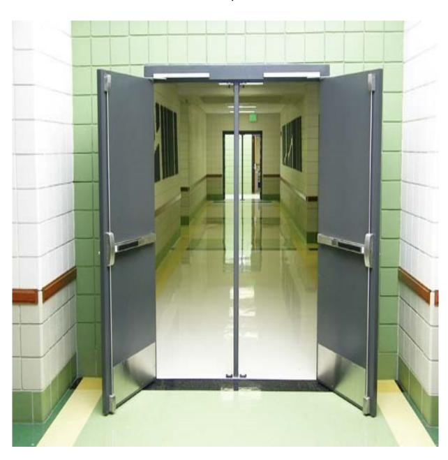
Any guess why wood doors would fail but not hollow metal? Fire rated applications with wood doors are only allowed 1/8" clearance. Having a pair of wood doors be nice and plumb and square with only a 1/8" gap is pretty tough.
