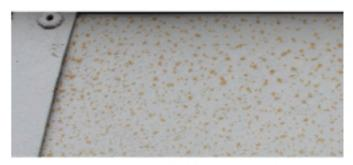
Rust generally forms on a door from the inside out. Once you see rust on the outside of a door then the core has been compromised.
