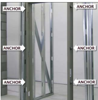
Proper anchor spacing
