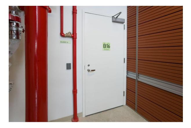
Fire doors and assemblies are a critical part of a building's passive fire protection system. The International Building Code (IBC) is the most widely-used building code in the U.S., and references NFPA 80 for the installation of fire door assemblies.
